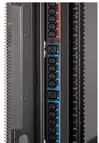
ePDU G3 mounted at 90-degree angle
